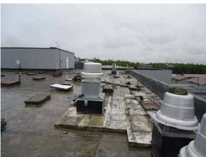
Roof B Wasilla, AK
