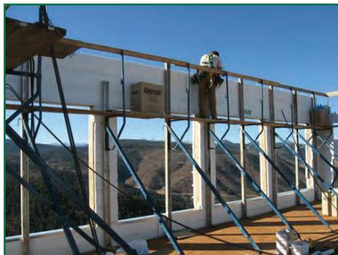
The construction of the main floor was relatively simple compared to the extraordinarily difficult foundation phase. The walls, which are twelve feet tall, have numerous large windows to utilize the abundance of natural light and capture the stunning views. They also provide support for the second story.
